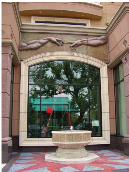
Hands 16 feet across in Forton MG with metal powder. This has been in place for about seven years and looks the same as when installed.
